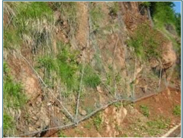
Steel Rope used to armour the mesh and fix the net at the toe of the
