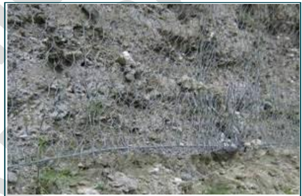
Steel Rope used to fix the net at the base of the slope
