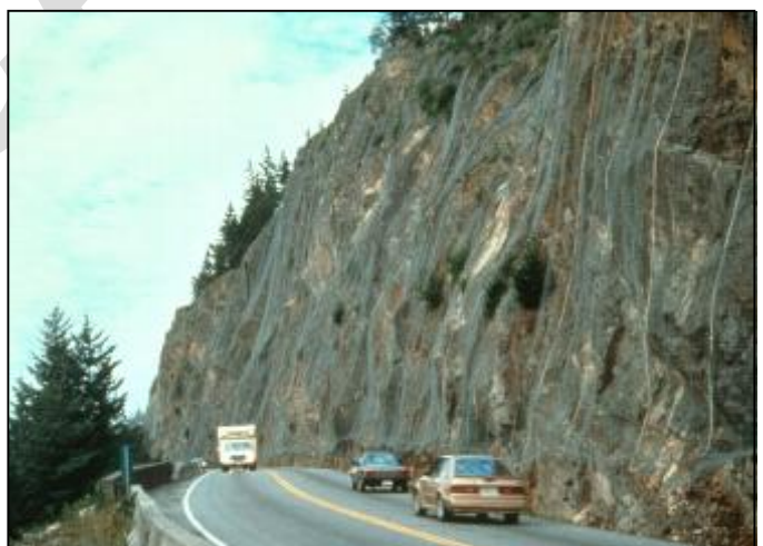
Example of Rockfall protection netting
