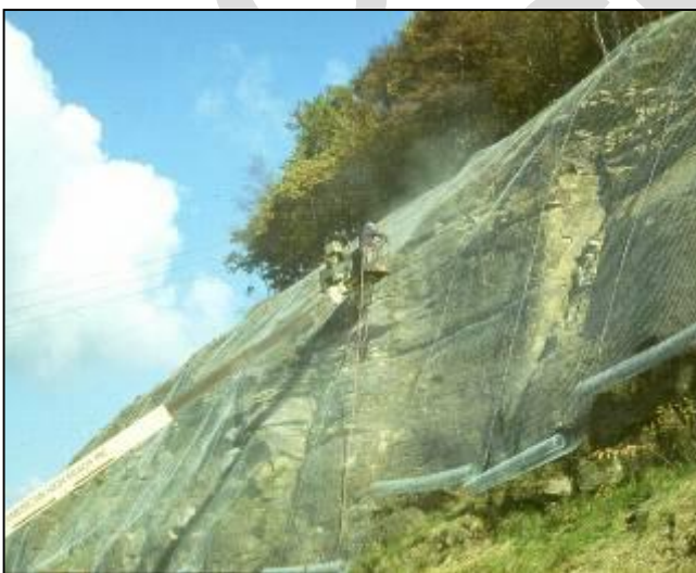
Example of Rockfall protection netting
