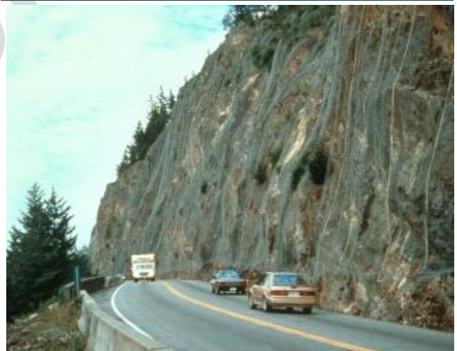
Example of Rockfall protection netting
