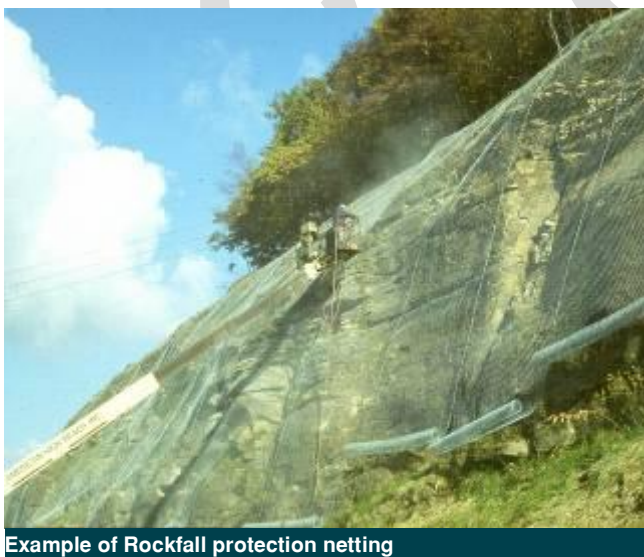
Example of Rockfall protection netting
