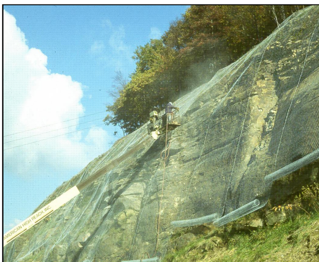
Example of Rockfall protection netting
