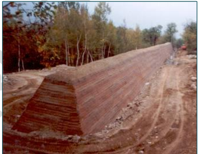
Rockfall Protection Embankment application
