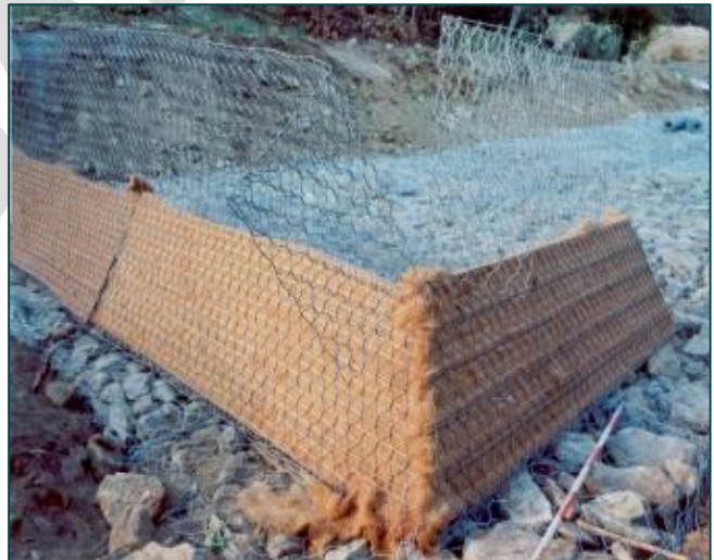
Rockfall Protection Embankment terminal
