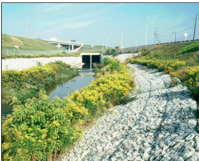
Example of Reno mattresses
